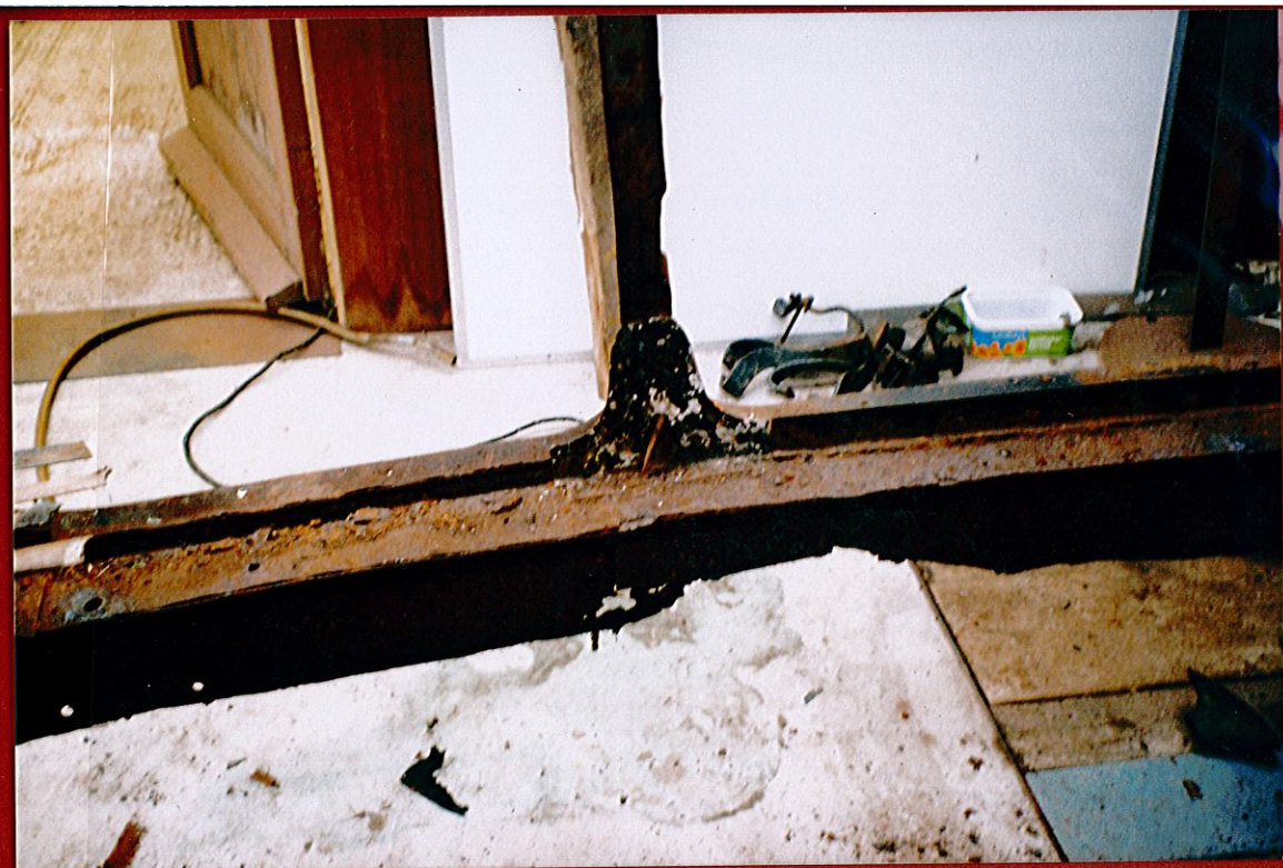
Memo Remains of sill Memo Bulkhead and chasis
